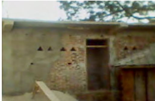
Figure School Toilet after monitoring
