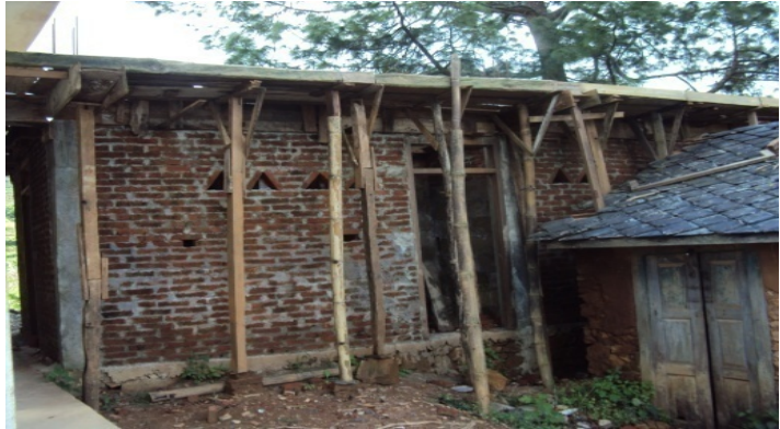
School toilet before monitoring, Dhading
