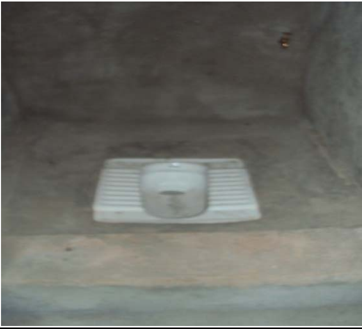
Completed School toilet
