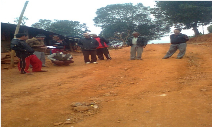
Monitors are monitoring of Jhagare road, Dhading
