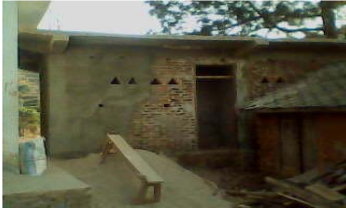
School toilet after monitoring
