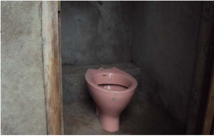
Completed School toilet
